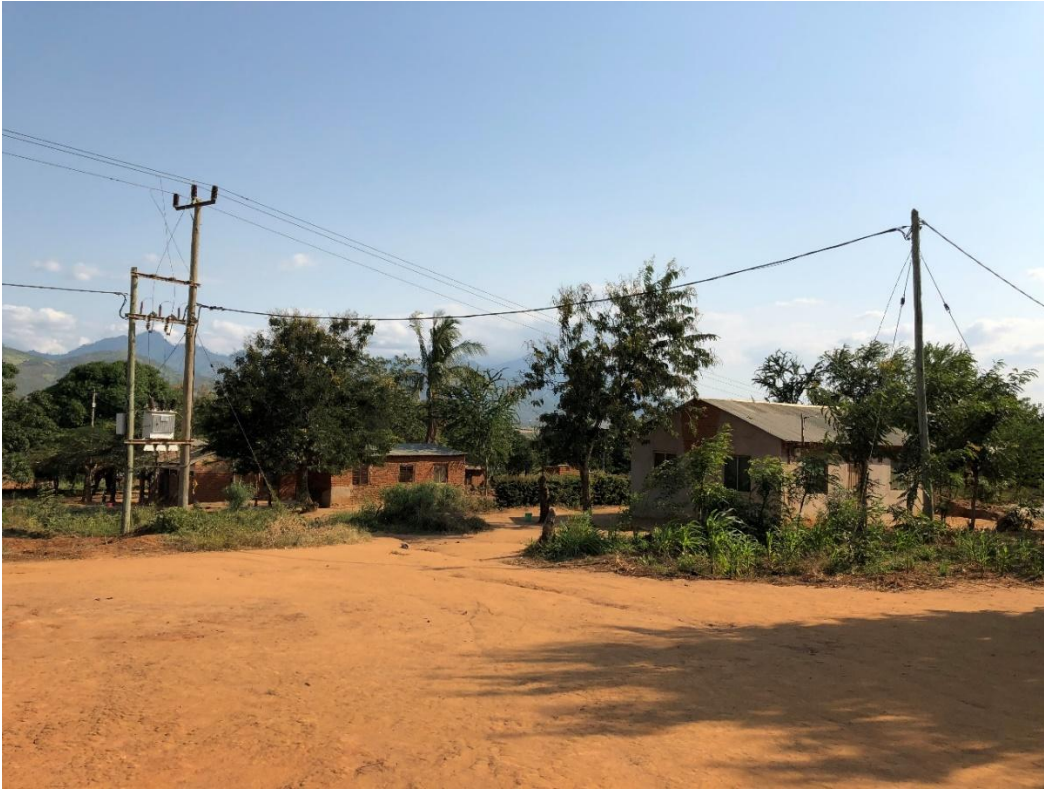
Fig: Example of national grid connection in Tanzania.
